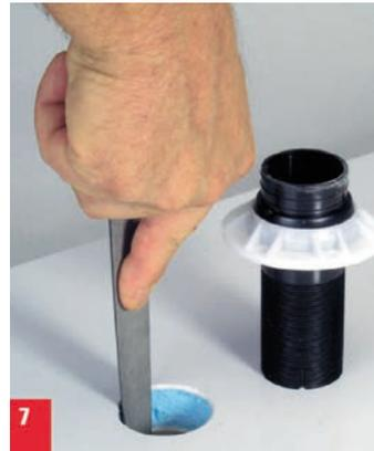
7. File the hole out. Insert the roof duct.
