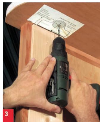
3. Put the template on the ceiling and drill a centre hole. For the template, go to *Template*, p. 7.
