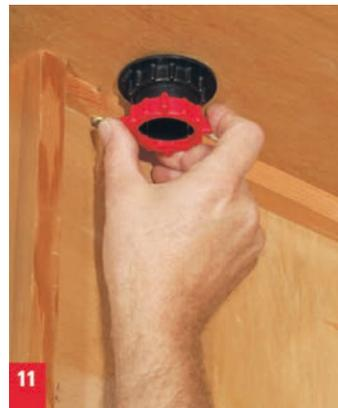
11. Carefully screw on the cone nut.
