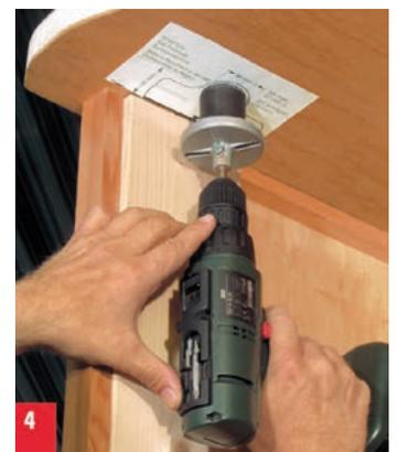
4. Use the circular drill bit to drill a hole of  $\text{Ø } 38$  mm from below.
